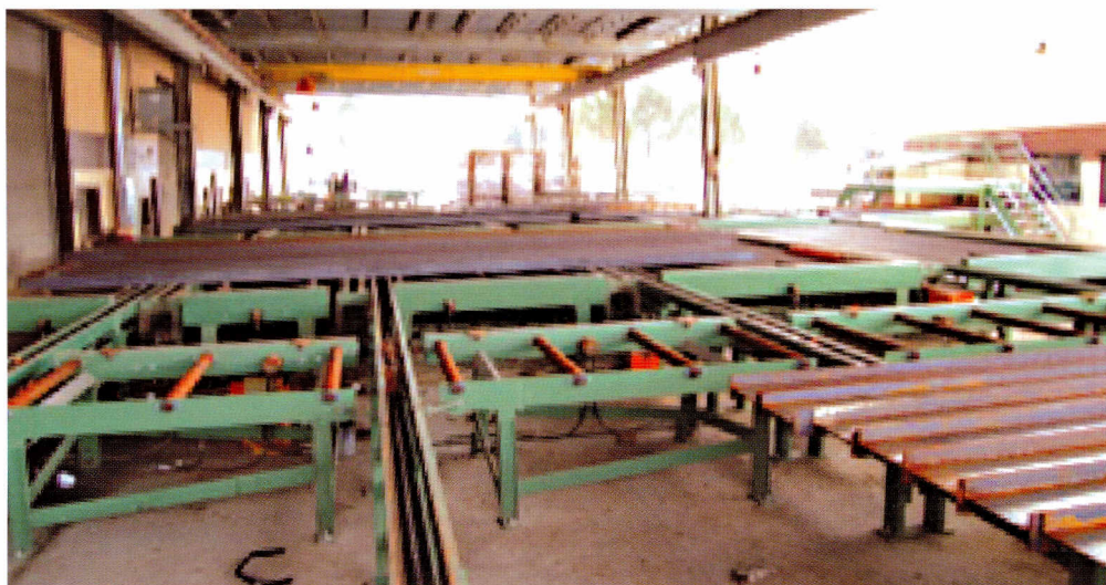
An effective material handling system, observed on a Peddinghaus tour, gives us efficiency to fabricate many sections in one day.
